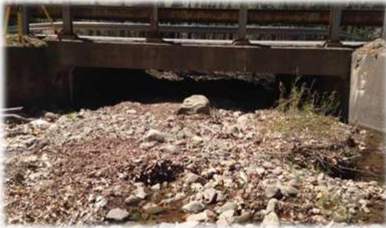
Flooding has been observed by the community at the location where Bungalow Brook crosses through a culvert under Claryville Road. The flooding in the Bungalow Brook area appears to be caused by flow from Bungalow Brook backing up at Claryville Road. A TR 55 analysis of flood discharges at Bungalow Brook was completed to determine peak flows:
