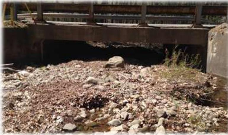
Flooding has been observed by the community at the location where Bungalow Brook crosses through a culvert under Claryville Road. The flooding in the Bungalow Brook area appears to be caused by flow from Bungalow Brook backing up at Claryville Road. A TR 55 analysis of flood discharges at Bungalow Brook was completed to determine peak flows:
